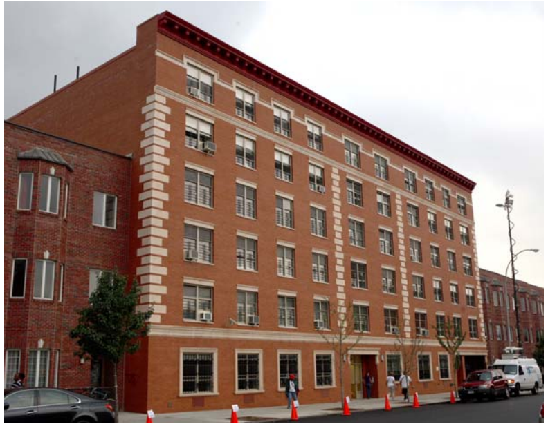
Myrtle Avenue Apartments was awarded the 2nd Energy Star label for high-rise residential buildings in the country.
