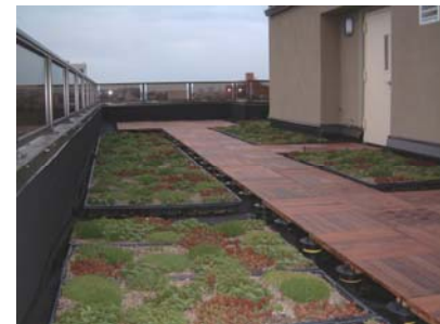
Green Grid Roof
